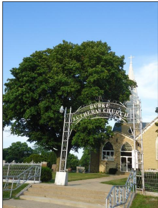
Burke Lutheran Church is and will continue to be a recognizable place within the community, photo courtesy Mead & Hunt, Inc. 2013
